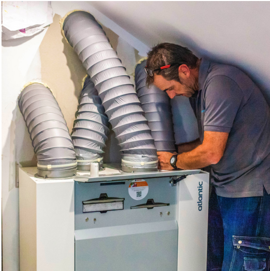
Raccordement de la VMC double flux !
